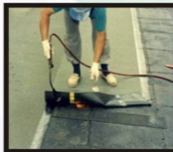
Position and flaming the bottom of surface
