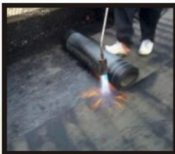
Position and flaming the bottom of surface
